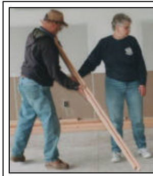
Bob and Mary Ann Hirn are cleaning up the interior of the Country School Museum in preparation for School Tours where a Nurse will be presenting home remedies that were used in years gone by. You can see the dry walling work and the electrical outlets that the Boys have installed.
