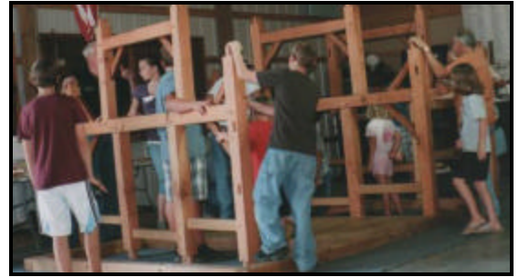
The young barn builders quickly learned that it really does take teamwork to successfully build a barn.
