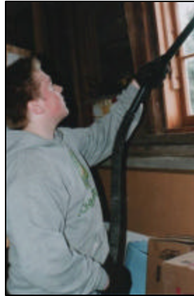
Jack Hill's grandson, Zack Hughes of Sandusky, is pictured vacuuming the webs out of the windows in the granary in the southwest corner of the Barn.
