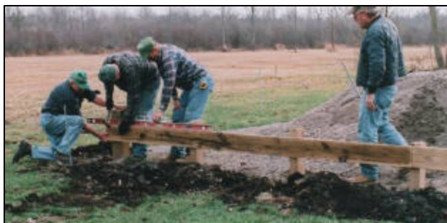
Pictured are Howard Gehrls, Wayne Lenton, Bob Hirn & George Wilson working on the foundation for the Sugar Shack that is just south of the Grain Elevator Building and another of the buildings that will be a part of our Village. They are installing the treated lumber foundation to support the rough sawn lumber building and act as a retaining wall for the stonecrete floor.
